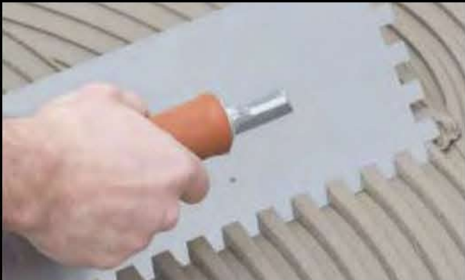
1. Cement laying on Floor
