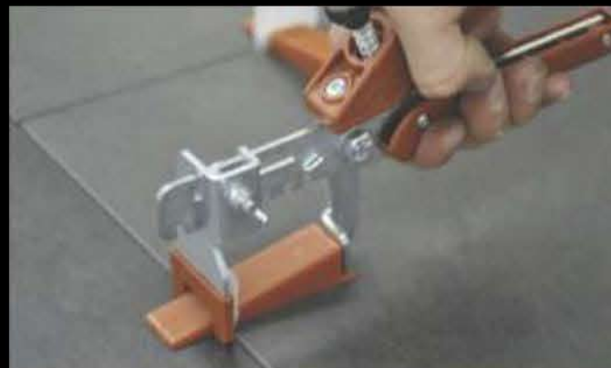
4. Levelling Wedges
