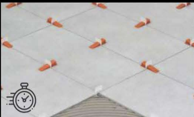
5. After Levelling Process leave it for 8-10 hrs.
