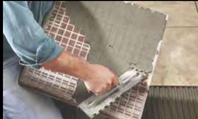
2. Cement laying on Tile
