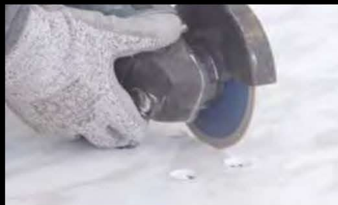
2. Cut with Diamond Blade Angle Grinder
