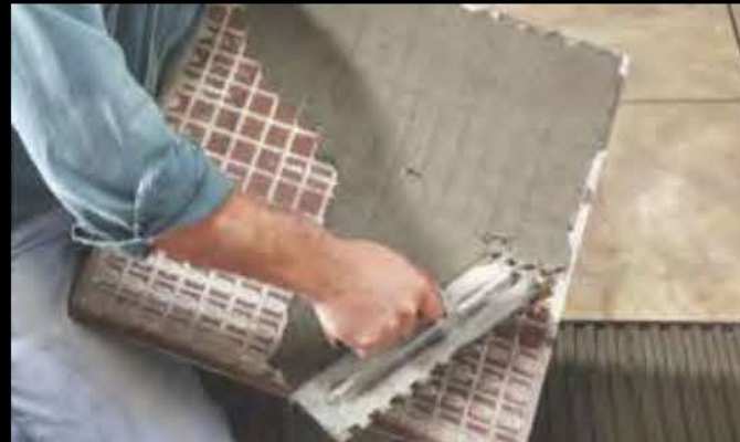
2. Cement laying on Tile
