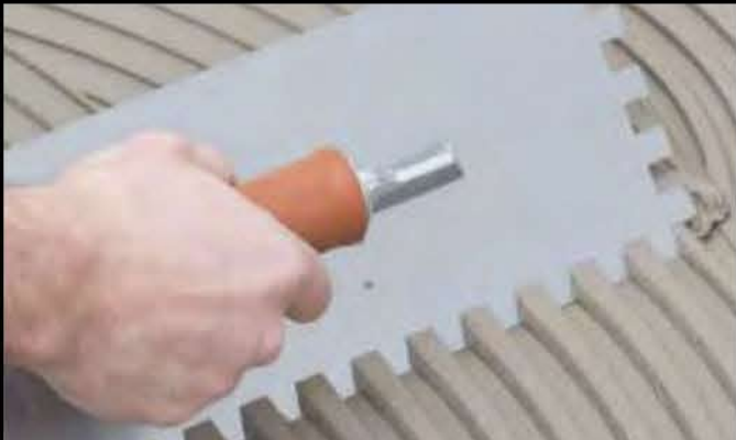
1. Cement laying on Floor
